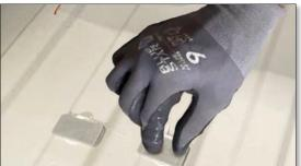
Please note: you only have approximately 20 minutes from beginning the gluing process untill till the floor has to be in place, all depending on the temperature and the humidity.
